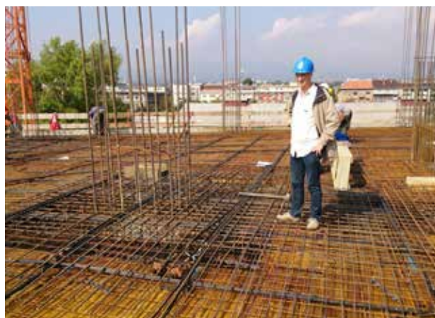
Figure 4. Reinforcement and unbonded tendons (smaller tower)
