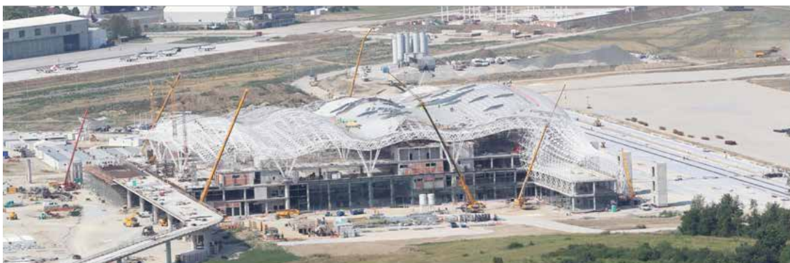
Figure 11. View of the roof structure
