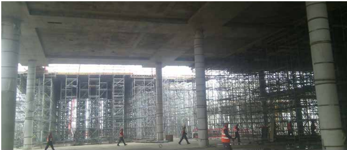
Figure 9. A view on the first floor slab with span 14.4x14.4 m, middle zone, columns height 10 meters thru two levels
