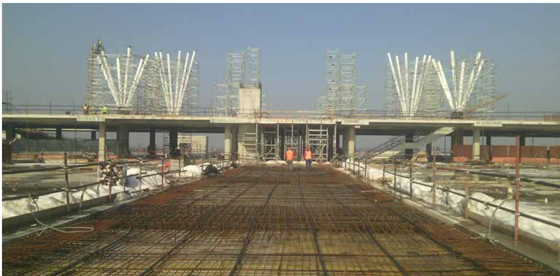
Figure 10. Pouring strip zone before monolithization
