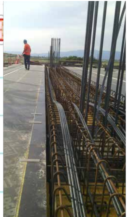
Figure 7. Tendons on parterre slab
