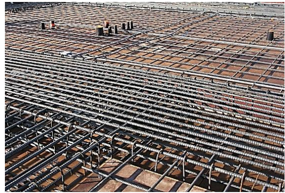
Figure 1. Conventional Reinforced Concrete Monolithic Slab System
