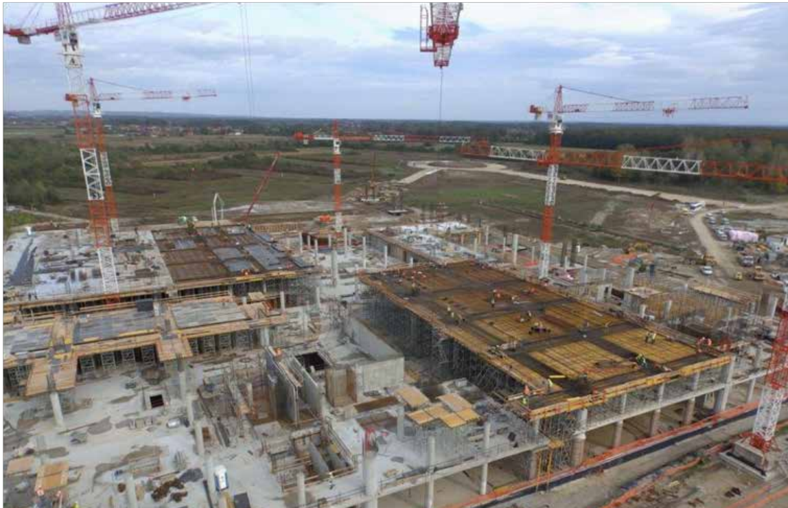
Figure 8. View of the building site from one of six cranes
