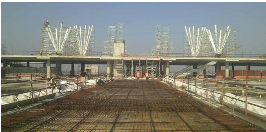
Figure 10. Pouring strip zone before monolithization
