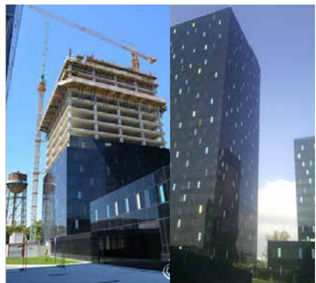
Figure 2. View of the taller tower during construction and the finished phase
