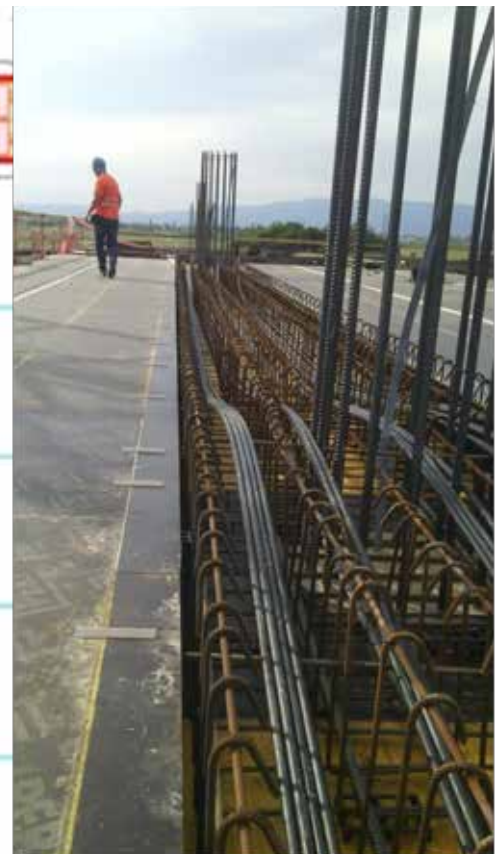
Figure 7. Tendons on parterre slab
