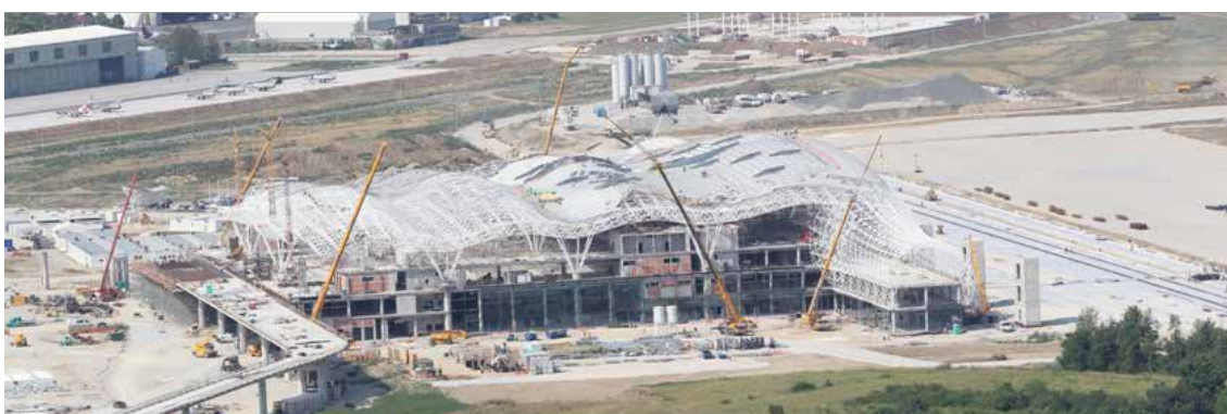
Figure 11. View of the roof structure
