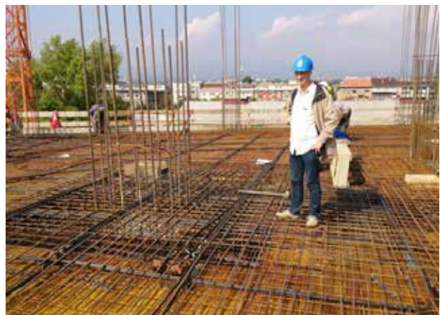
Figure 4. Reinforcement and unbonded tendons (smaller tower)
