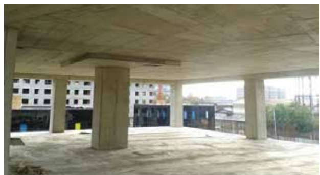
Figure 5. View on a slab after removing of the formwork (smaller tower)
